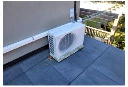
Refrigerant Lines: repair/replace insulation
