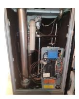
Filter: basement and 3rd level air-handler -replace 1-per-6 to 12 months
