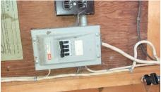
GFCI: provide to exterior outlet
