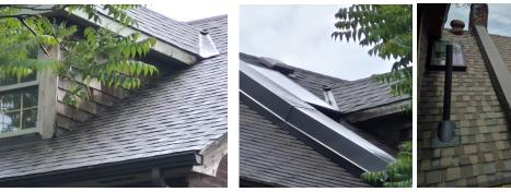
2nd Flat: overall surface in good repair Flat Surface: mostly not visible, parapet at southeast leaking (stain in ceiling)- requires maintenance/ flashing - minor repair overall
