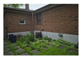
\*\*Lot Grading: low areas around foundation: re-grade away from house \*\*Walk(s): seal gaps along foundation wall
