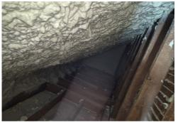
FLOORS/WALLS rear extension: low to grade- more prone to moisture damage, presently do not suspect and appears well sealed, monitor
