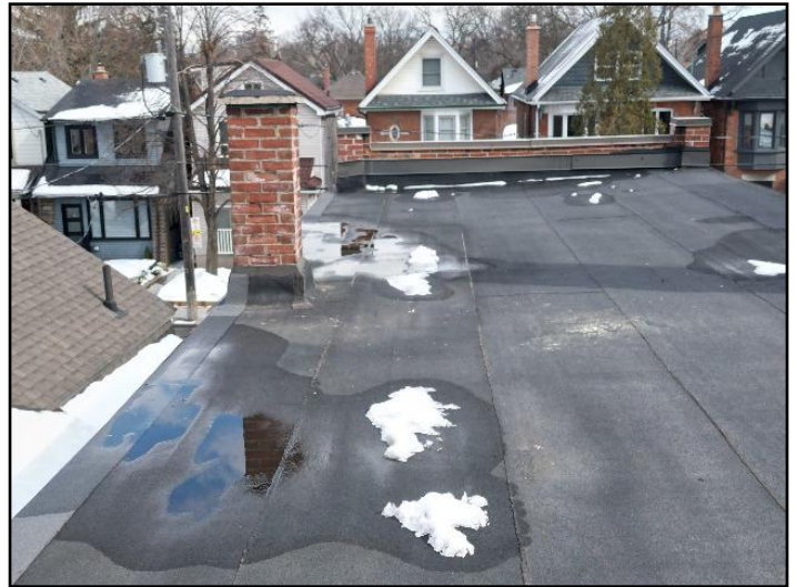
Modified bitumen membrane
