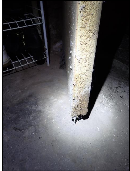
Absorption line, MDF door (absorbant)
