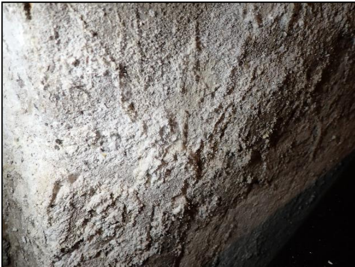
Efflorescence
