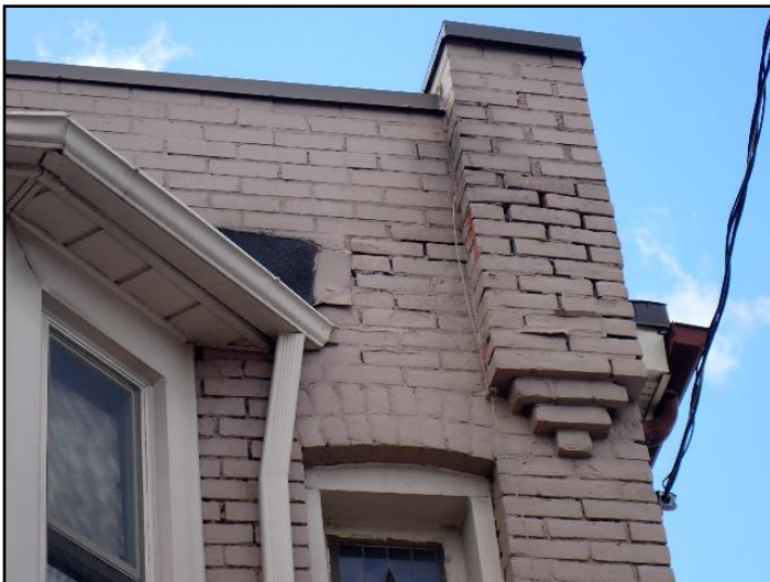
Mortar deterioration
