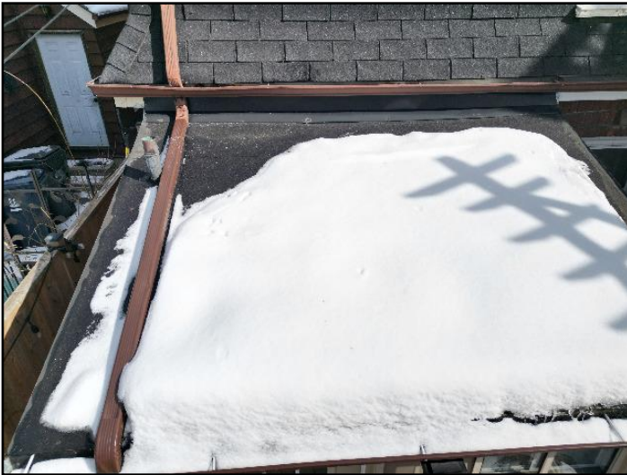
Modified bitumen membrane
