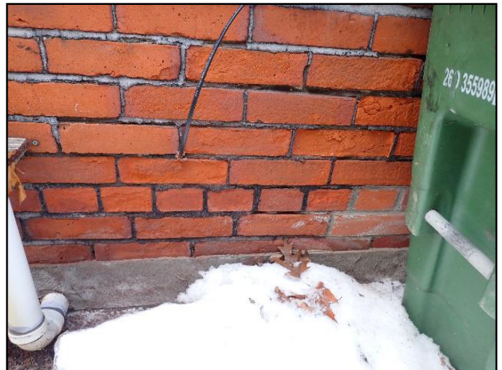
Mortar deterioration
