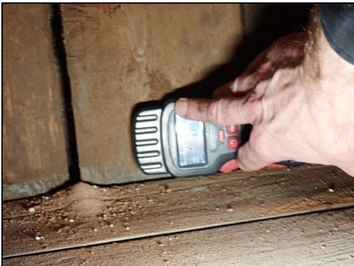
Typical reading noted - Dry
