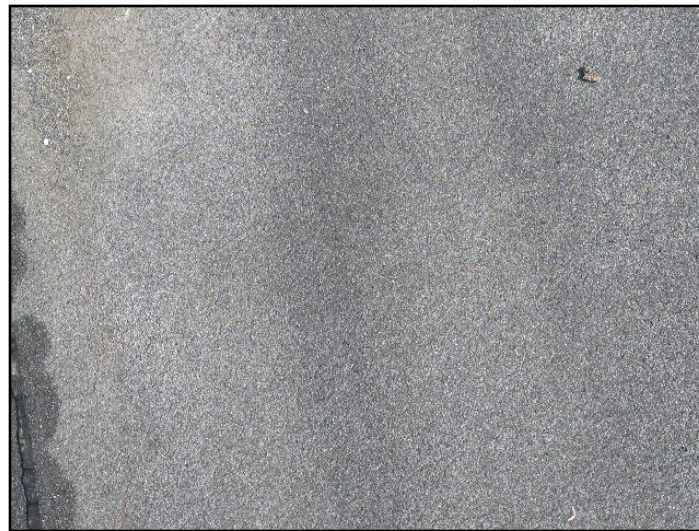
Modified bitumen membrane
