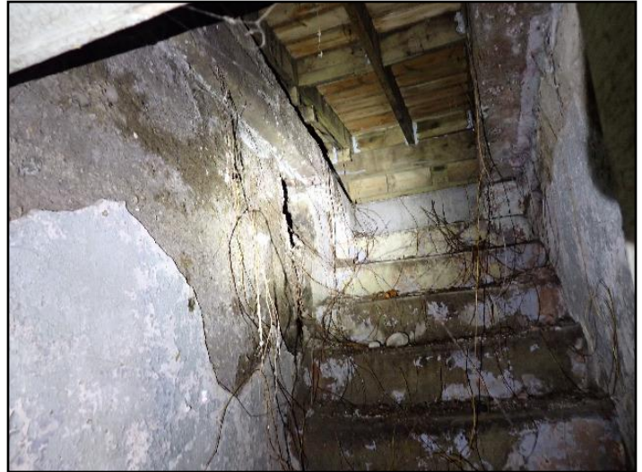
Walls - spalling
