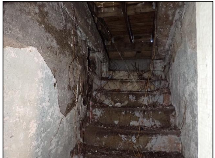
Crumbling concrete(outside)
