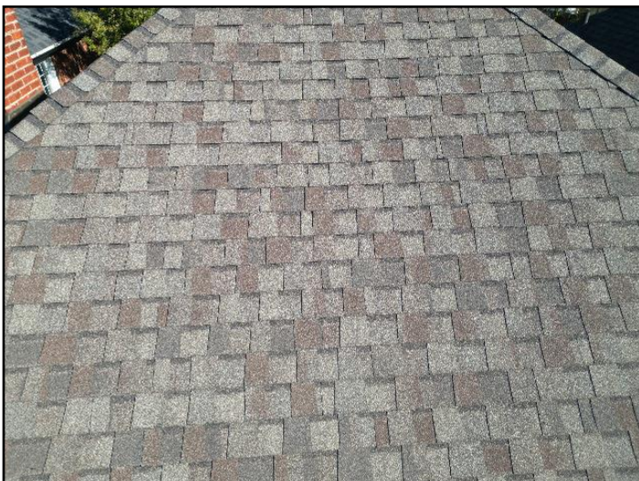
Asphalt shingles
