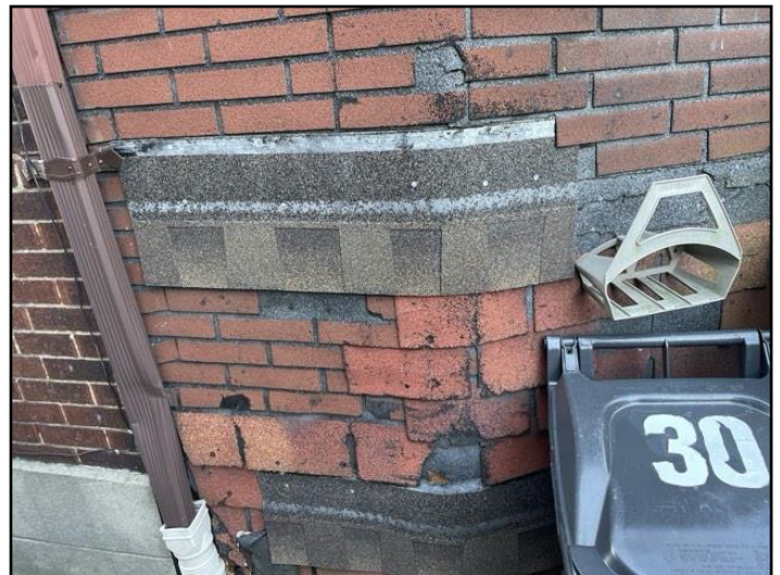
Deteriorated shingles
