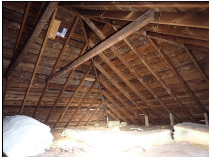
Rafter, roof joists, plank sheathing
