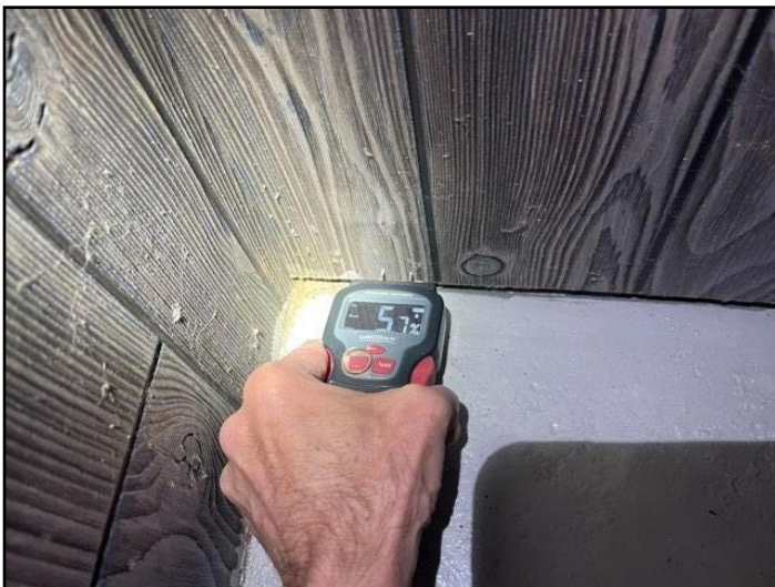
Right (viewed from street) [Interior Rm. Wall]
