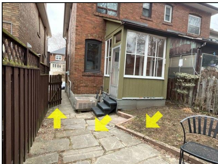
Lot Grading - Ensure slope away from home
