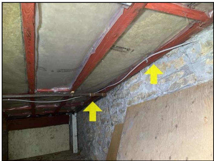
Deck Connection quality: Inspect annually
