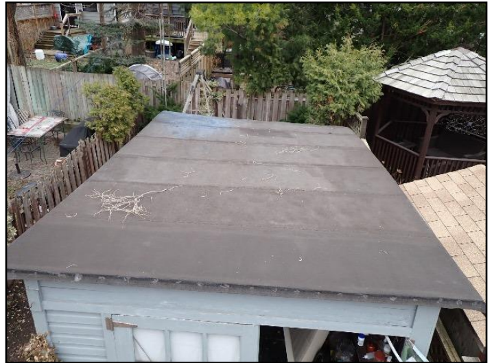
Modified bitumen membrane
