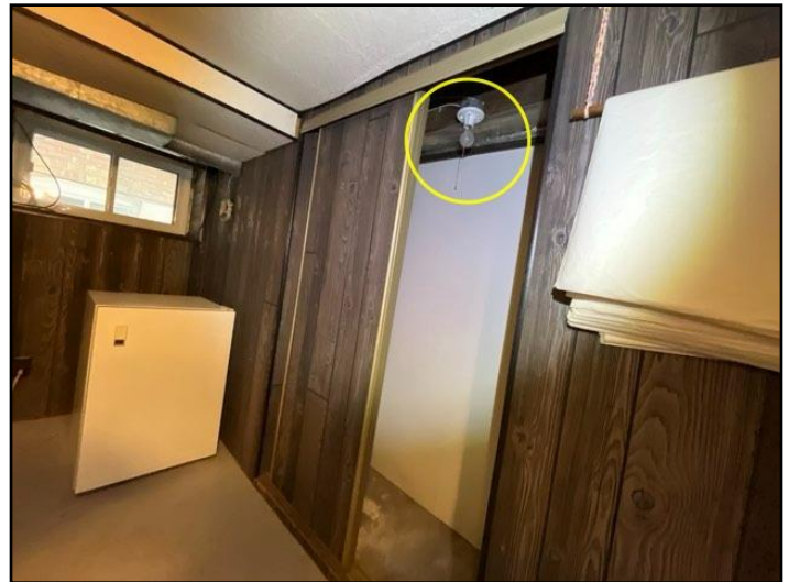
Exposed bulbs: Example, Front Basement
