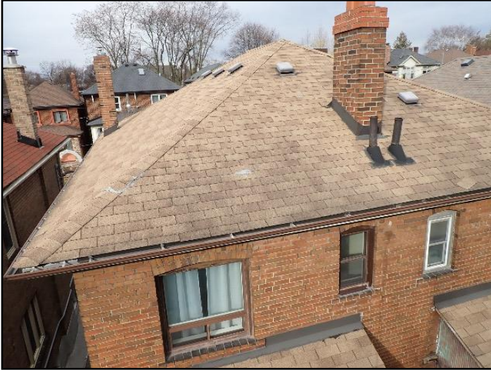
Asphalt shingles: Rear
