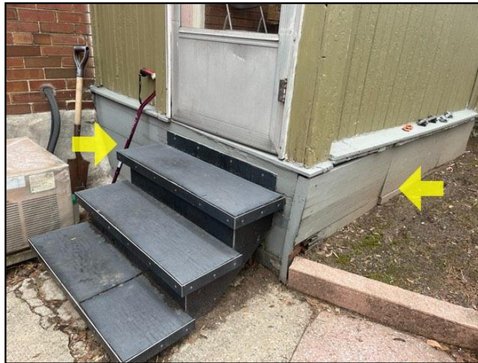
No access was gained to the crawlspace
