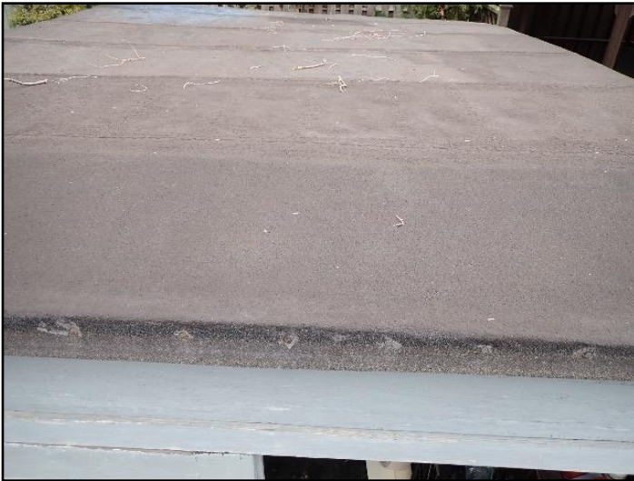
Detail: Modified bitumen membrane
