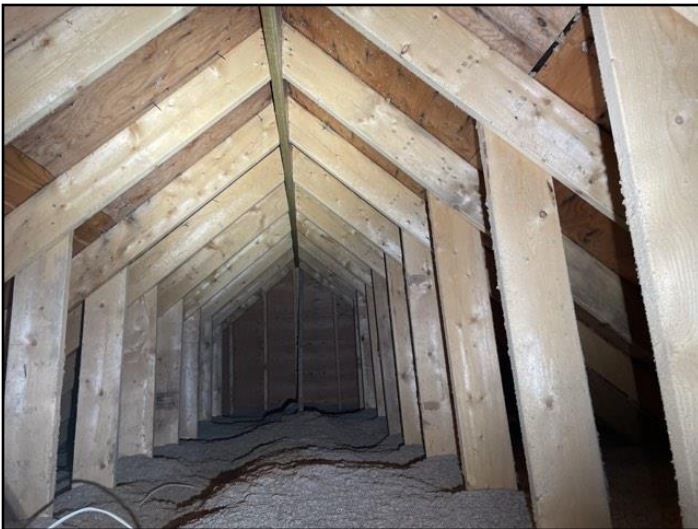
Rafters / Joists / Plywood sheathing
